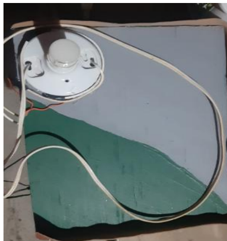
Fig -2: Electrical indication system of the seismic sensor Source: Analysis of the investigation
